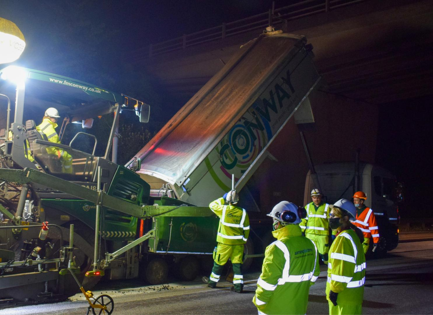
The innovations used in developing the new materials have driven substantial carbon savings. The high RAP content resulted in a 23% reduction in carbon compared with traditional materials, while manufacturing the asphalt as a warm mix saved a further 14% as it only had to be heated to 150°C. Standard hot mix asphalts are heated to 180°C.
