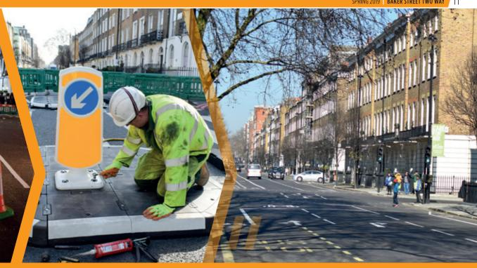
Matt continues: "The term maintenance team installed over 100 road signs in advance of the works. These signs would eventually direct the traffic following the switch to two-way running. To avoid any confusion before this point, the signs were covered with stickers which would be removed during the final steps of the switchover. We needed to test how long this would take so that we could factor it into our schedule and synchronise the different teams on site."
