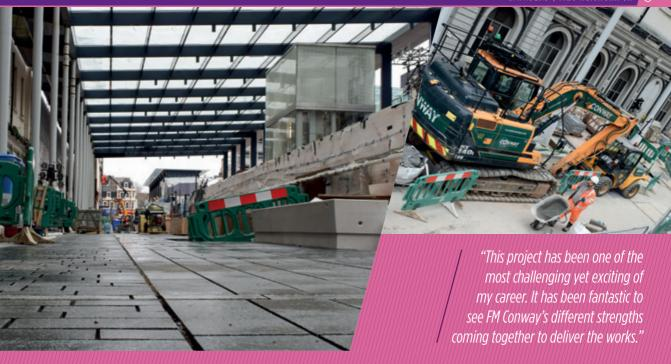
station. Being mindful to minimise the load on the tunnel and station infrastructure below ground, the team capped these services with a lightweight expanded clay material, specially imported from Norway, to backfill up to the formation level. This was followed by 3,000 tonnes of FM Conway's recycled type-1 sub-base mix and a jointed reinforced concrete slab base.
