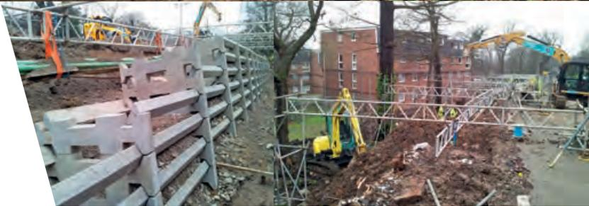
"We looked at options for a like-for-like brick replacement, as well as feasibility for strengthening some of the sections. But we developed a completely different approach using interlocking concrete blocks that was ultimately cheaper, more robust, and more attractive. The 'green wall' was comfortably the best option for residents – and the efficiency savings meant major benefits for the project as a whole."
